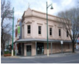
B5661 Campbell Connelly Building
