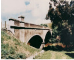
B2841 Fyansford Bridge Hamilton Hwy
