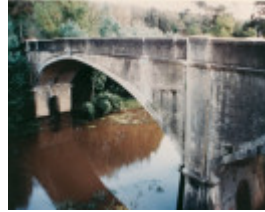
B2841 Fyansford Bridge Hamilton Hwy
