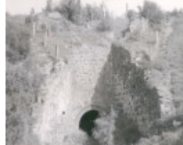
B1637 Lime Kiln Limeburners Point Geelong
