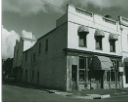
B5102 Former List's Building
