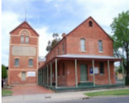
B5717 Friedrich & Bassemir Bakery Buildings
