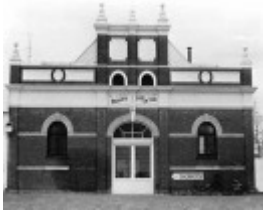
B3914 Fuse Factory
