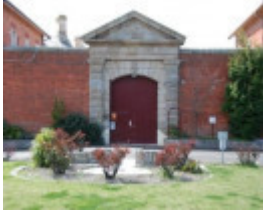
B1369 Gaol Entrance & Walls
