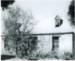
B1850 Former Travellers Rest Inn
