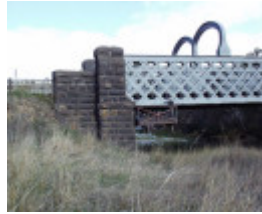
B1541 Redesdale Bridge
