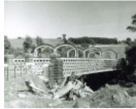
B1541 Redesdale Bridge
