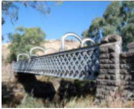
B1541 Redesdale Bridge
