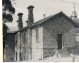
B1854 Original Police Barracks
