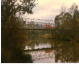
B6852 Queens Park Bridge North Side
