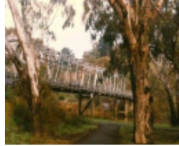
B6852 Queens Park Bridge Geelong
