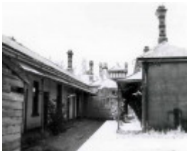
B3978 Servant's Quarters
