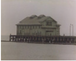
B5643 Yarra Pier Cargo Shed
