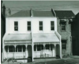
B3910 Terrace Houses
