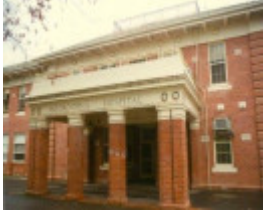
B6773 Entrance Portico
