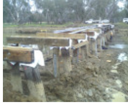
B7031 Murchison Rail Trail Bridge sub structure 2010
