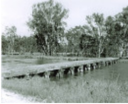
B7031 Murchison rail bridge
