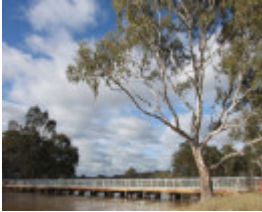
B7031 Murchison Rail Trail bridge 2010
