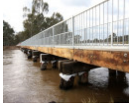
B7031 Murchison Rail Trail bridge 2010
