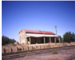
1 manangatang railway station complex wattle street manangatang rear view
