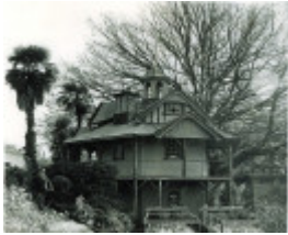
B3942 Former Office Forest Commission Nursery
