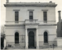
B1051 Fmr E S & A Bank Fraser St Clunes
