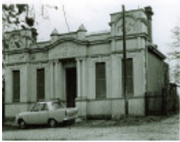
B5844 Former Creswick Shire Hall
