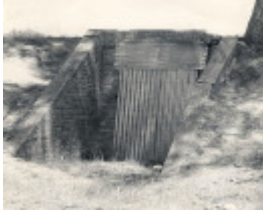
B2343 Railway Store Creswick
