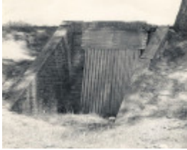
B2343 Railway Store Creswick
