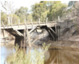
B7067 Jeparit bridge abutment
