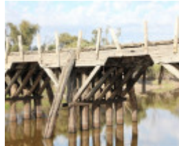
B7067 Jeparit bridge piers
