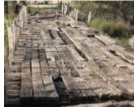
B7067 Jeparit bridge deck
