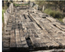
B7067 Jeparit bridge deck
