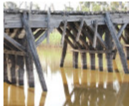
B7067 Jeparit bridge piers
