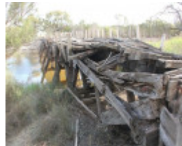
B7067 Jeparit Bridge 2011
