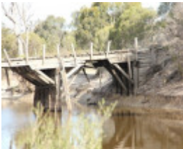
B7067 Jeparit bridge abutment
