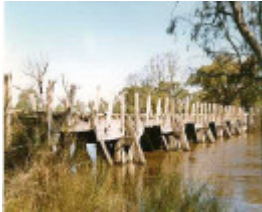
B7067 Jeparit Bridge
