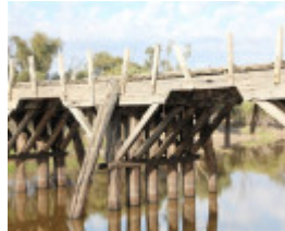
B7067 Jeparit bridge piers
