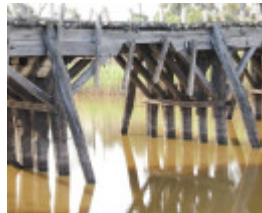
B7067 Jeparit bridge piers
