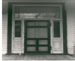
B1805 Rosebrook front Doorway
