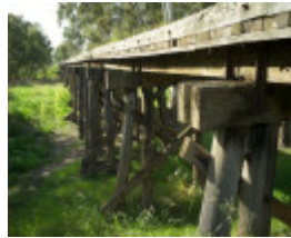
B6910 Wimmera River Rail Bridge
