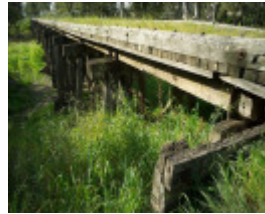
B6910 Wimmera River Rail Bridge
