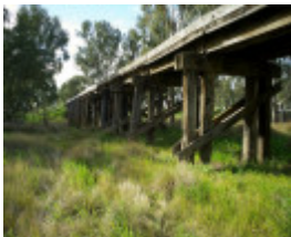
B6910 Wimmera River Rail Bridge
