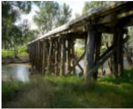
B6910 Wimmera River Rail Bridge
