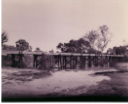
B6910 Wimmera River Rail Bridge
