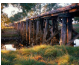
B6910 Wimmera River Rail Bridge
