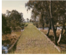
B6910 Wimmera River Rail Bridge
