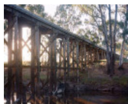
B6910 Wimmera River Rail Bridge
