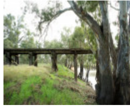
B6910 Wimmera River Rail Bridge
