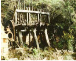
B3218 Nine Mile Creek Historic Place
