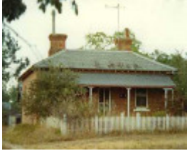
B4498 Former Police Residence
