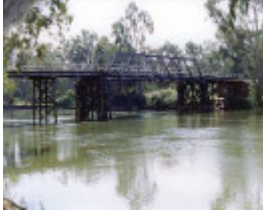
B6803 Howlong Truss Bridge
