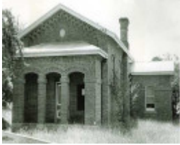
B1705 Court House Yackandandah
