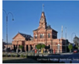
B2722 Court House & Post Office
