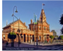
B2722 Court House & Post Office
