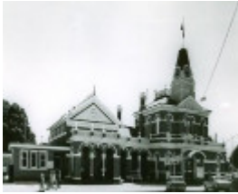
B2722 Court House & Post Office
