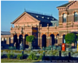
B2722 Court House & Post Office
