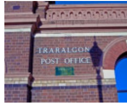
B2722 Court House & Post Office
