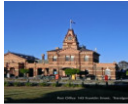
B2722 Court House & Post Office
