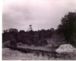
B6954 Tyers Road Bridge
