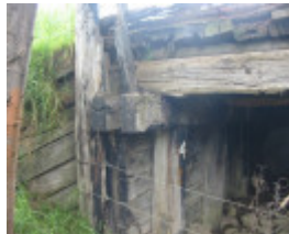
B6954 Tyers Road Bridge abutment
