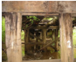
B6954 Tyers Road Bridge piers
