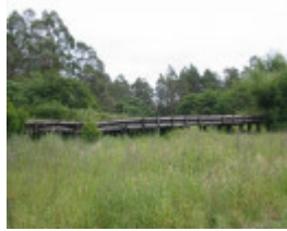
B6954 Tyers Road Bridge
