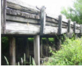
B6954 Tyers Road Bridge
