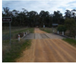
B6835 Kingower Bridge deck
