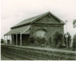
B5319 Goods Shed, Riddell's Creek station
