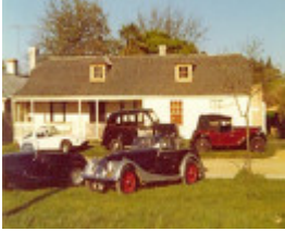
B4383 57 Aitken Street
