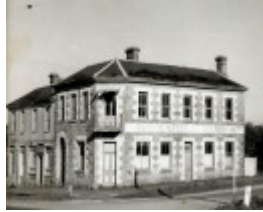
B1493 Former Hotel Malmsbury
