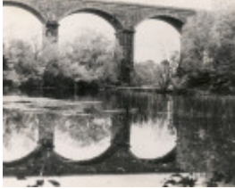
B1288 Railway Bridge Malmsbury
