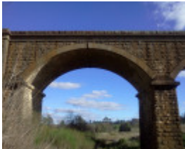
B1288 Malmsbury viaduct detail
