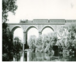
B1288 Railway Bridge over Coliban River
