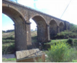
B1288 Malmsbury viaduct 2011
