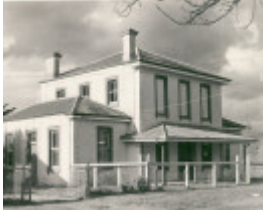
B2086 Former Court House & Police Station
