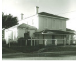
B2086 Former Court House & Police Station
