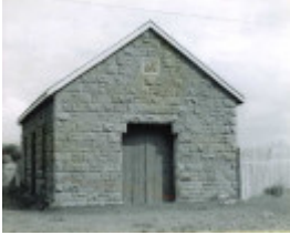
B1855 Bluestone Building Daylesford Rd Malmsbury
