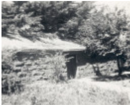
B2407 Original Rear of House
