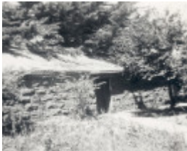
B2407 Original Rear of House
