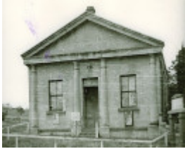
B0306 Former Malmsbury Town Hall
