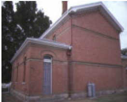
mansfield court house rear elevation feb1985
