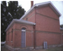
mansfield court house rear elevation feb1985
