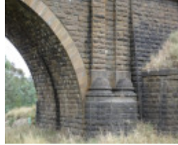
B2681 rail bridge over Riddell's Creek detail
