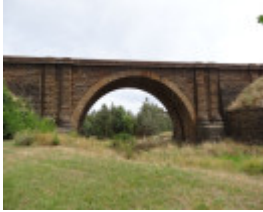
B2681 rail bridge over Riddell's Creek
