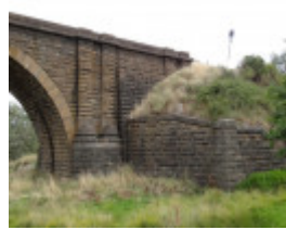
B2681 rail bridge over Riddell's Creek
