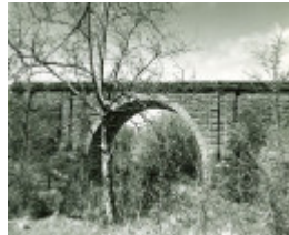
B2681 Rail Bridge Over Riddells Creek
