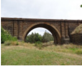
B2681 rail bridge over Riddell's Creek
