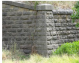
B2681 rail bridge over Riddell's Creek wall detail
