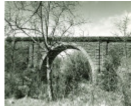
B2681 Rail Bridge Over Riddells Creek
