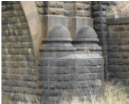
B2681 rail bridge over Riddell's Creek detail.
