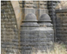
B2681 rail bridge over Riddell's Creek detail.
