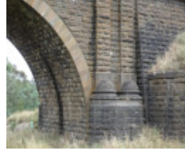
B2681 rail bridge over Riddell's Creek detail
