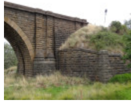
B2681 rail bridge over Riddell's Creek
