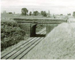
B4646 Road Bridge Malmsbury
