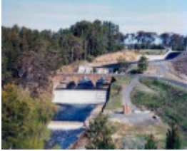
B6766 Upper Coliban Spillway Bridge
