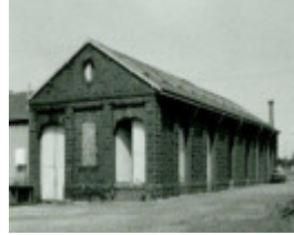
B3847 Kyneton Railway Station Goods Shed
