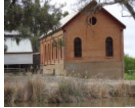
B3577 Psyche Bend pump house
