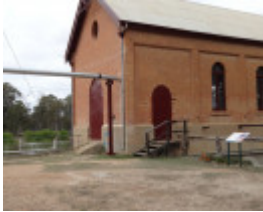
B3577 Psyche Bend pump house
