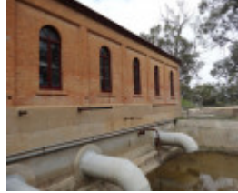
B3577 Psyche Bend pump house
