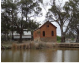
B3577 Psyche Bend pump house
