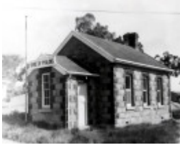
B1782 Shire Offices Pyalong
