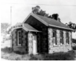
B1782 Shire Offices Pyalong
