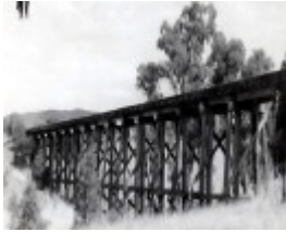
B3053 Railway Bridge
