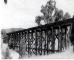
B3053 Railway Bridge
