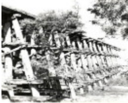
B3287 Railway Bridge Pyalong
