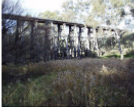
B3287 Railway Bridge Pyalong
