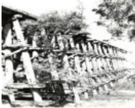
B3287 Railway Bridge Pyalong
