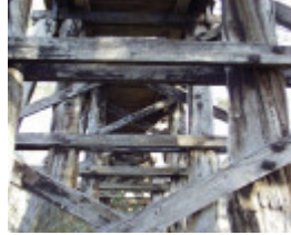
B3287 Railway Bridge Pyalong
