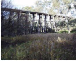
B3287 Railway Bridge Pyalong
