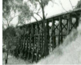
B3287 Railway Bridge Pyalong
