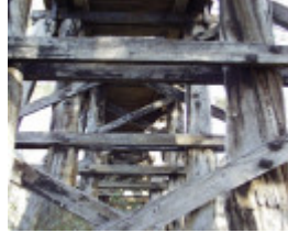
B3287 Railway Bridge Pyalong
