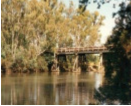
B6956 Old Hume Hwy Bridge
