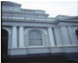
maryborough court house facade detail aug1984
